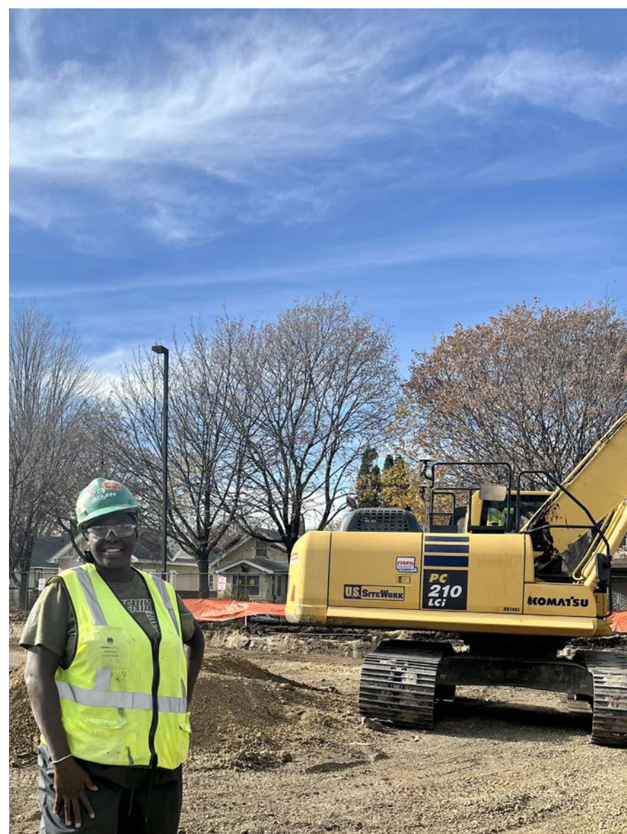
Ms. Delmarie Nelson, 51, on the NorthPoint construction site. Photo courtesy of NorthPoint Health & Wellness Center
