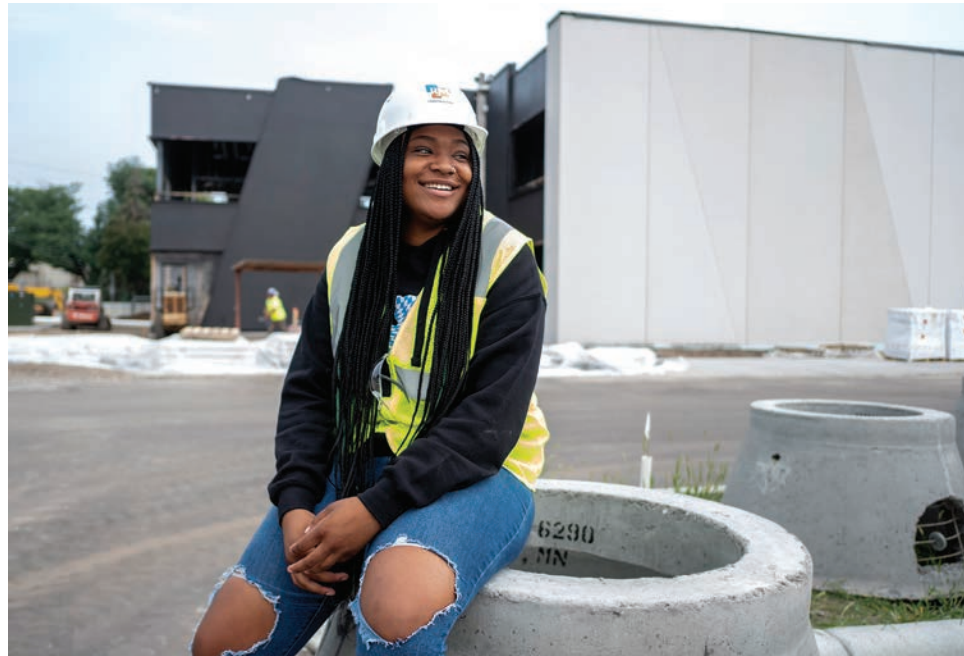
Ni’Kiyah Cotton’s summer just may turn into a construction career. Photo by David Pierini
